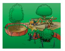
Instruct construction personnel to keep fencing intact and the fenced area clear of building materials, waste, and excess soil. No digging, trenching, or other soil disturbance should be allowed within the fenced area.
